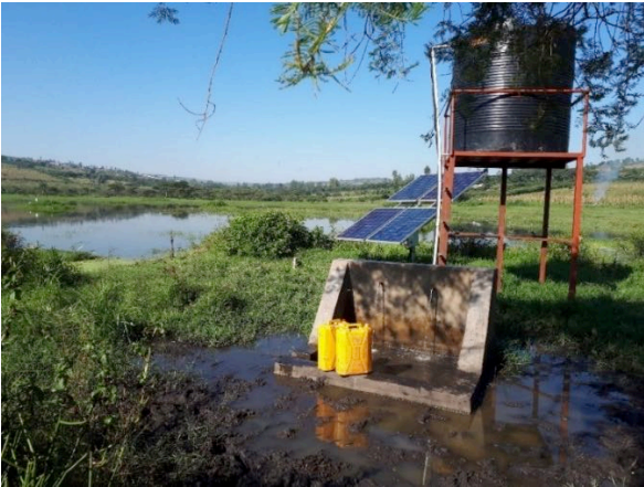
Figure 8. Small (Type B) sized piped systems with storage tanks
